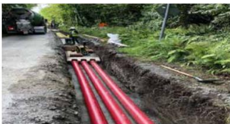
Figure 2-1 Typical 400 kV Cable trench
