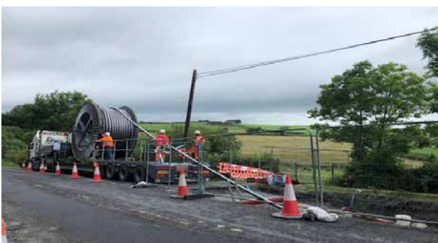
Figure 12: Cables being pulled into the ducts and jointing bay
