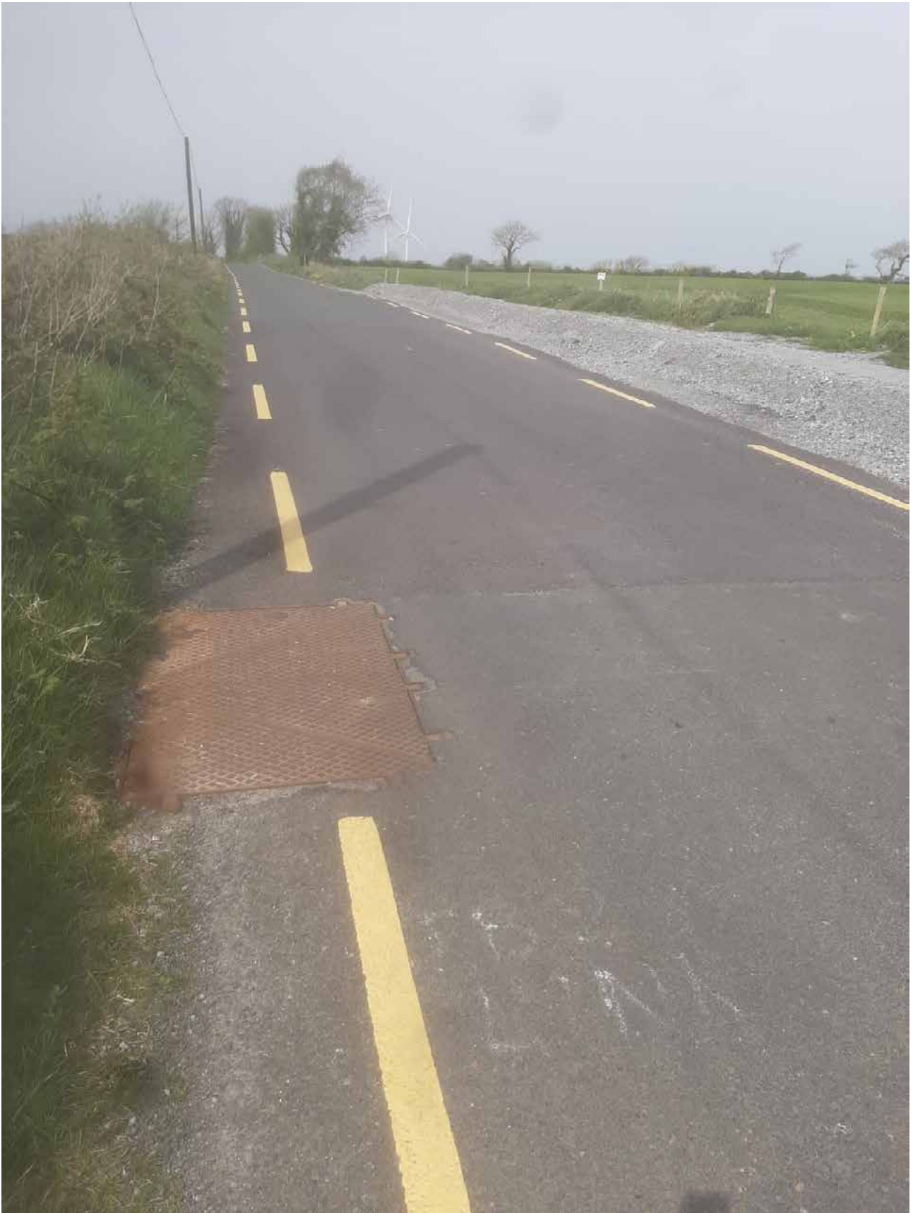
Figure 14: A typical road reinstatement
