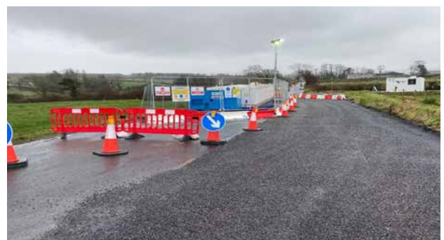
Figure 13: A typical passing bay in operation during cable jointing
