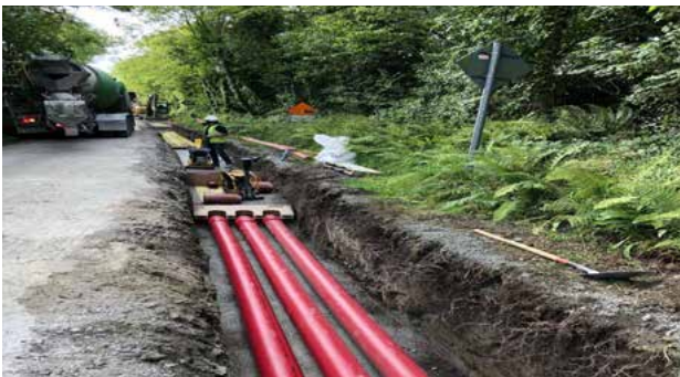
Figure 10: A typical cable duct installation in the road
