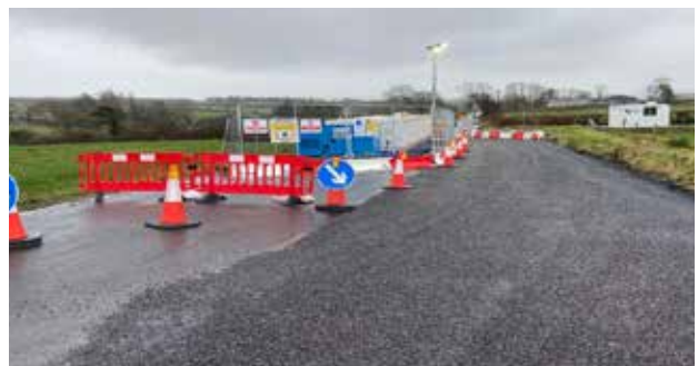
Figure 14: A typical passing bay in operation during cable jointing
