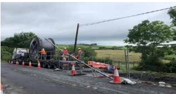
Figure 13: Cables being pulled into the ducts and jointing bay
