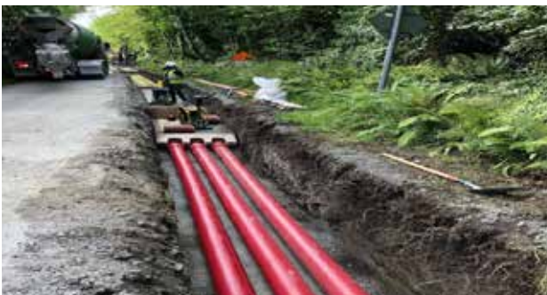
Figure 11: A typical cable duct installation in the road
